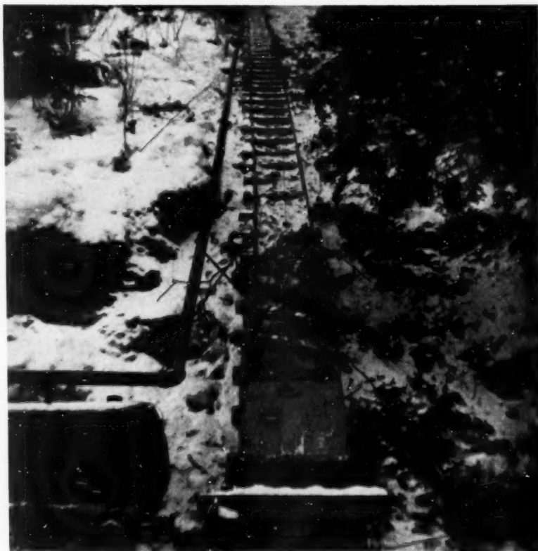
Inclined surface tram up the south slope of Rock Creek from the compressor level to the exploration adit level on American Alloy Metals, Inc.'s Ivanhoe claim.
